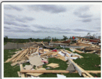
EF-4 damage to a home near Linwood, KS (NWS Survey).
